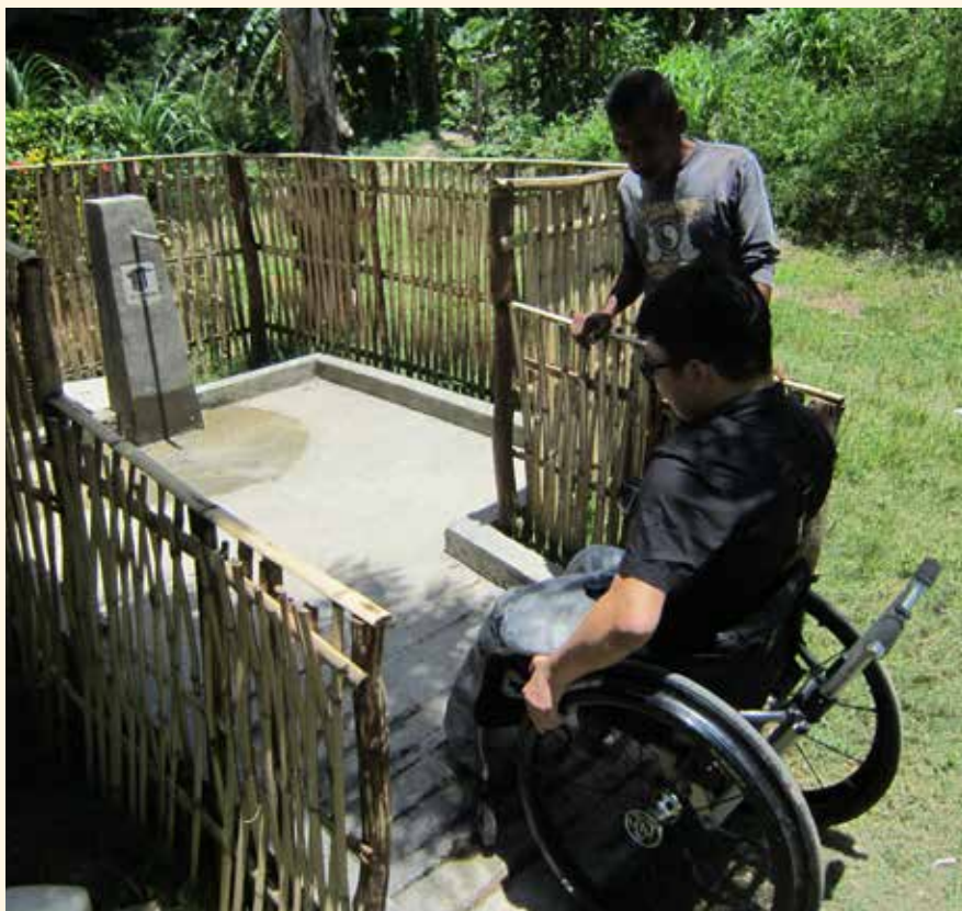
Huy Nguyen (Former WaterAid Australia Equity and Inclusion Officer) pictured, front, here demonstrating use of a newly constructed accessible water point in Liquica district.
